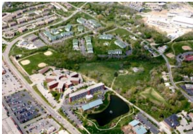
Looking Southwest to Callahan Hall
