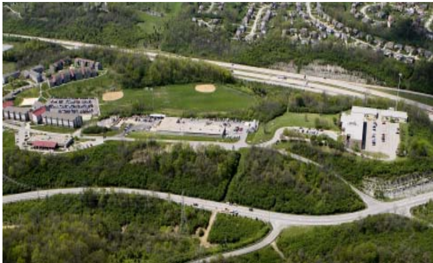
Looking West to North Village, Existing Maintenance Facility and Campbell Hall
