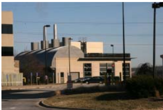
Existing Power Plant
