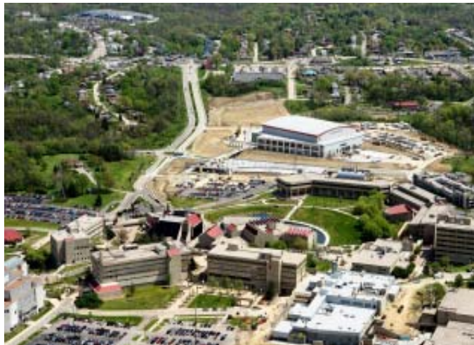
Looking East from Kenton Drive
