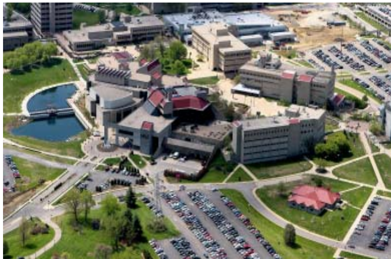
Looking Southwest to the Library and Central Receiving
